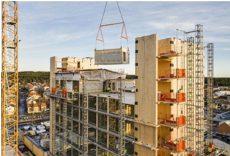
Mass timber is ideal for prefab modular construction [14]
