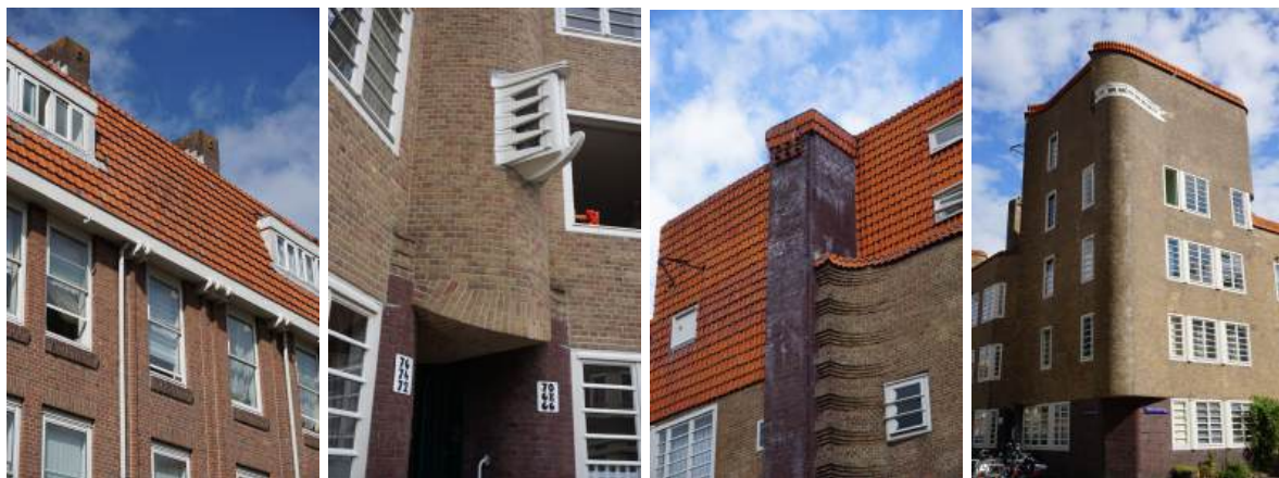
Subtle material and surface gestures enhance the larger formal gestures of De Dageraad. Soldier courses around thresholds, alterations in brick depth, and data marked by changes in brick color are essential gestures in the project.
